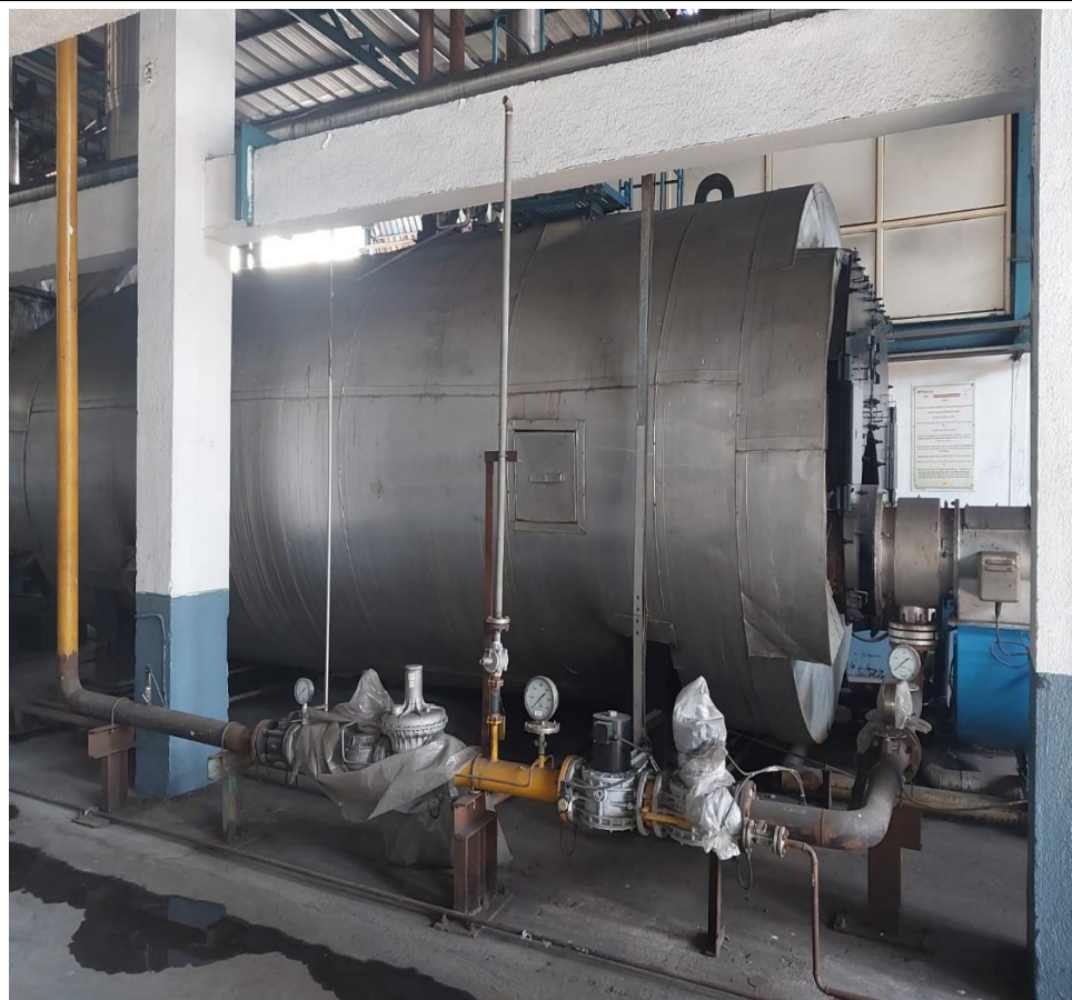
PNG metering Kit and consumer connection with PRV at Boiler
