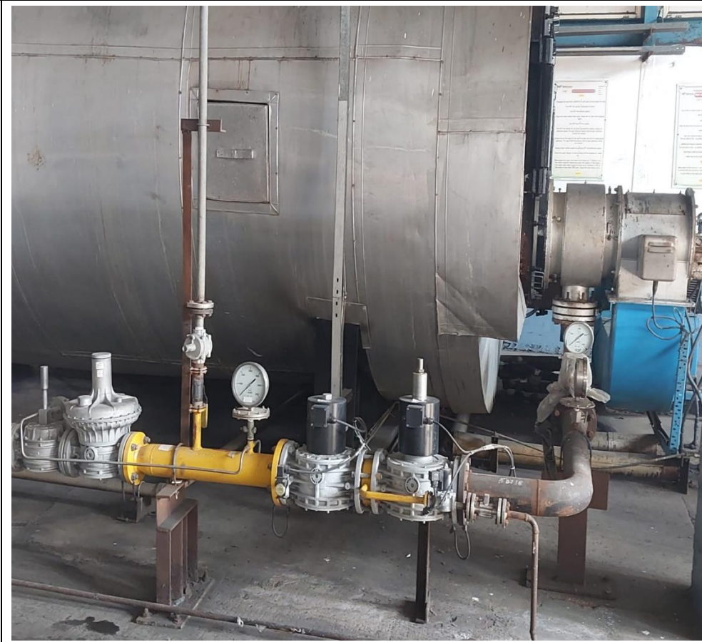
PNG metering Kit and consumer connection with PRV at Boiler
